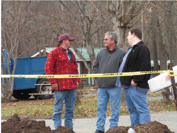
EBCI equipment operator Clarence Murphy, former Historic Sites Keeper Jerry Dugan, and THPO Russ Townsend discuss excavation process at an EBCI project site.
